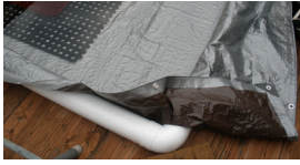
Detail of wash pit construction.
