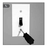
1. Loosen the screws of the wall-mounted switch plate.
